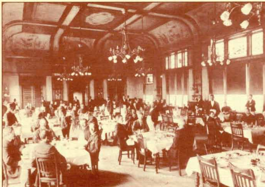
In this elegant restaurant in the old Granite Building, Sibley's operated a restaurant from 1893 until 1906, which attracted customers from as far away as Elmira and Corning. The Tower Restaurant in the Sibley's Building at Main Street and Clinton Avenue was successor to the Granite Building restaurant.
